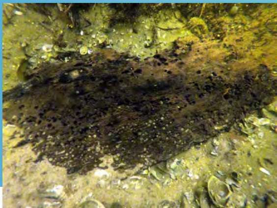
LEFT: An exposed timber shows marine worm damage and fastener holes
