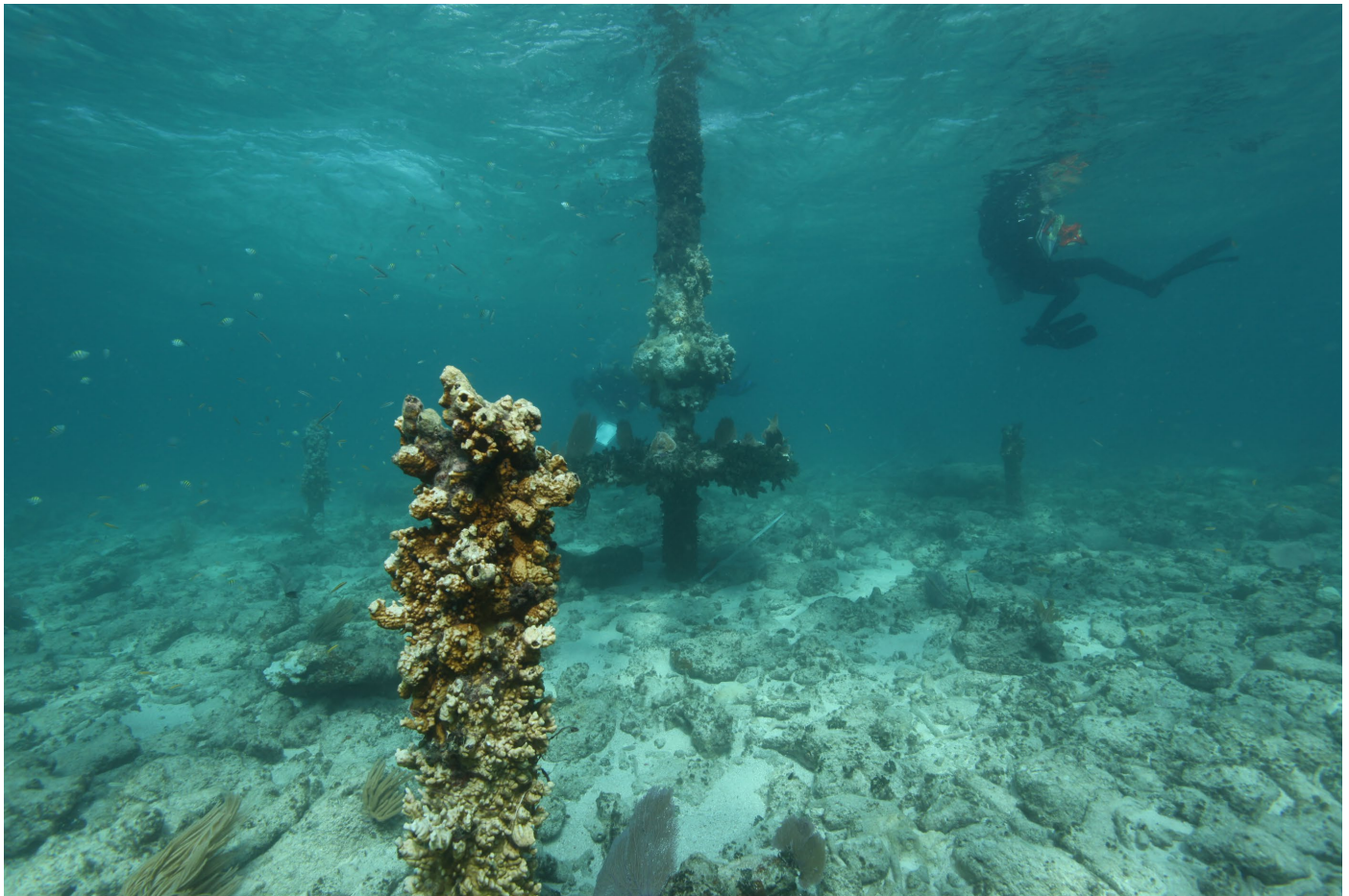
The beacon at American Shoal was bolstered by three stakes and a system of turnbuckles that helped it withstand storm wind and waves. Photo by Matthew Lawrence, NOAA
